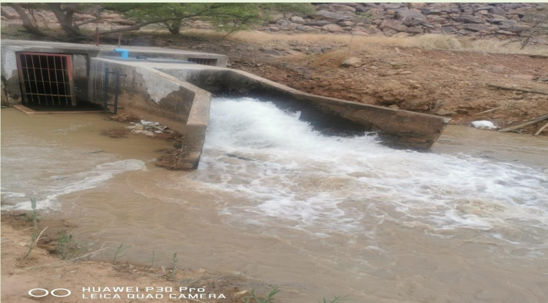
Picture ...: Replacement of control valve at fish eagle dam
