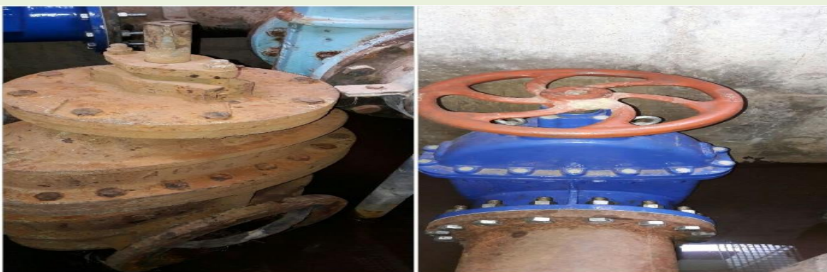
Replacement of old Valves at 7ML Reservoir
