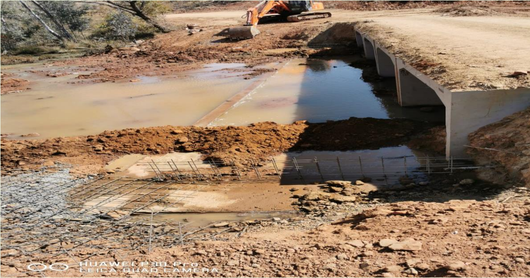
Picture ...: Rehabilitation of access road to the Warmbad Dam side
